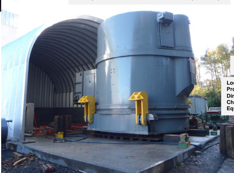
The transformer was offloaded to a storage plinth as a spare for the nuclear power station which involved rotating the transformer 90° to access storage building.
