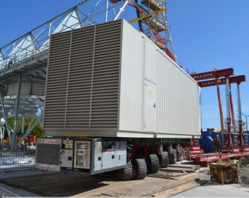
Once positioned on the plinth the hydraulic gantry lift system was used to lift the generator from the SPMT and place the generator to its operating position on the plinth.
